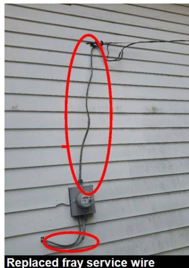
Replaced fray service wire
