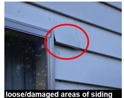
loose/damaged areas of siding
