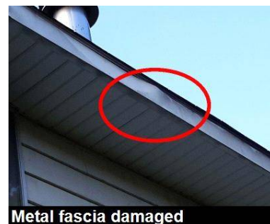
Metal fascia damaged
