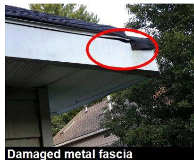
Damaged metal fascia
