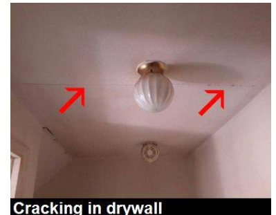
Cracking in drywall
