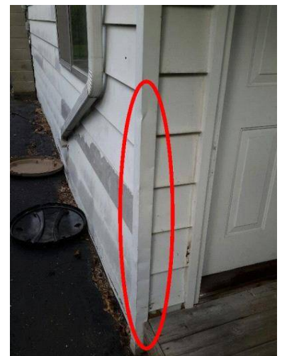
Damaged to metal corner piece
