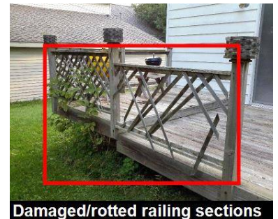
Damaged/rotted railing sections
