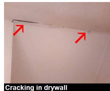
Cracking in drywall
