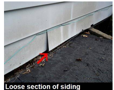
Loose section of siding
