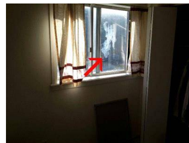
Bad seal, missing screen
