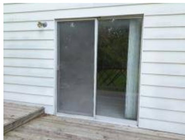
No casing around door
