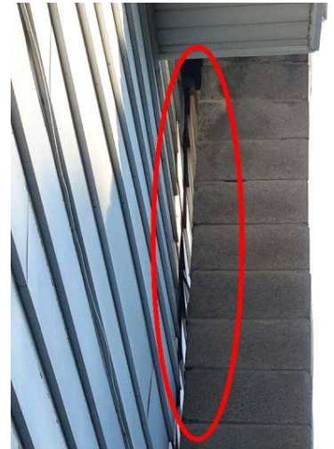
Chimney separating from house
