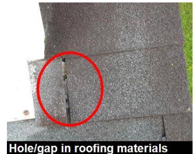
Hole/gap in roofing materials
