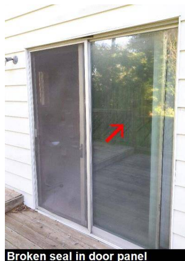
Broken seal in door panel
