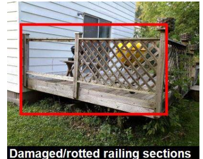
Damaged/rotted railing sections
