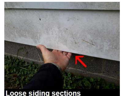
Loose siding sections
