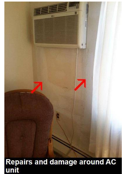
Cracking in drywall
