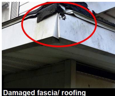
Damaged fascia/ roofing
