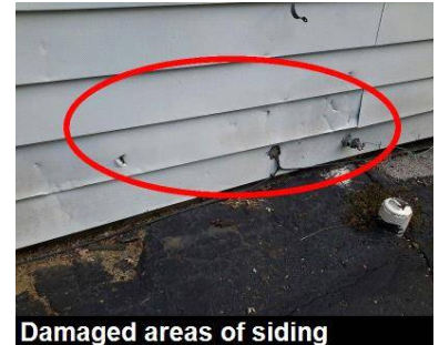
Damaged areas of siding
