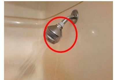
Small leak in showerhead
