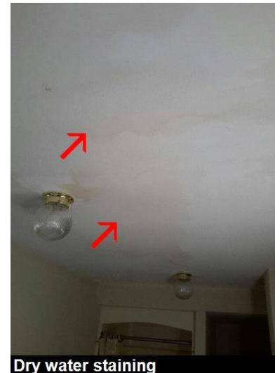
Dry water staining
