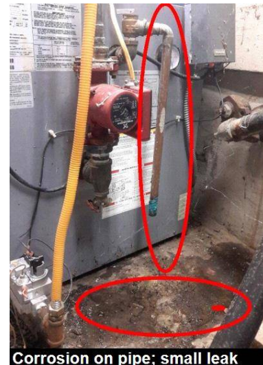
Corrosion on pipe; small leak
