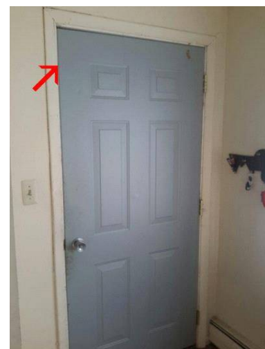
Binding noted at top of the door
