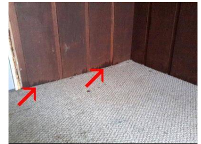
Water staining at bottom of wall
