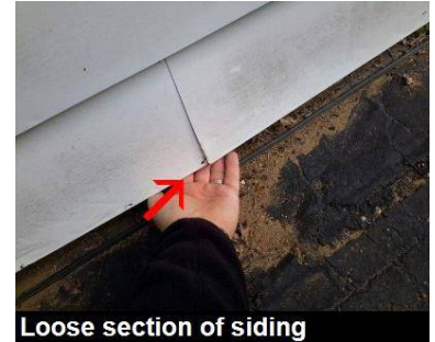
Loose section of siding
