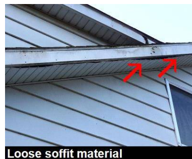
Loose soffit material
