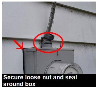
Replace frayed service wire
