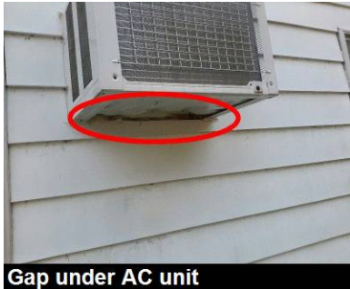
Gap under AC unit
