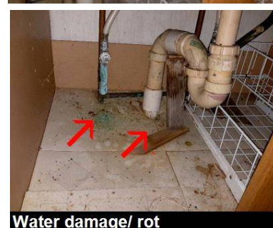
Water damage/ rot
