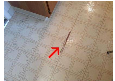
Damaged floor tile
