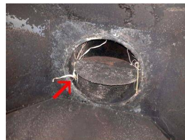
Nesting material in chimney stack
