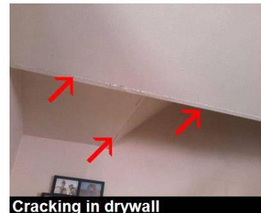
Cracking in drywall
