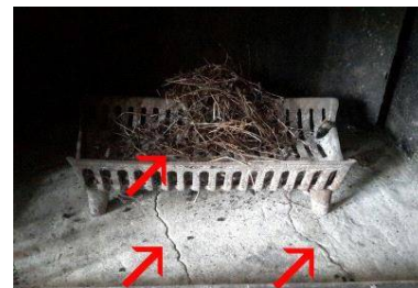
Cracks in cement; nesting material inside
