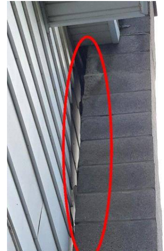
Chimney not secured to house
