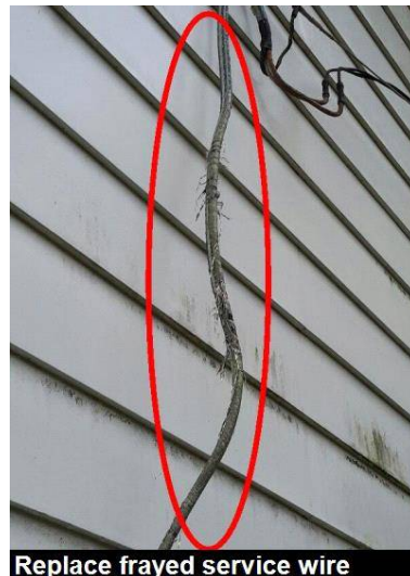
Replace frayed service wire
