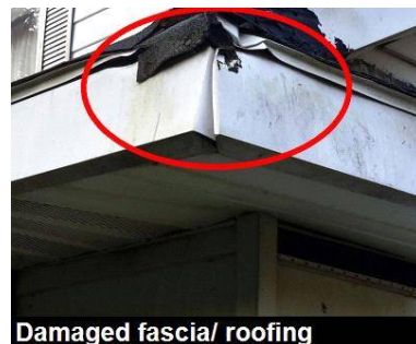
Damaged fascia/ roofing
