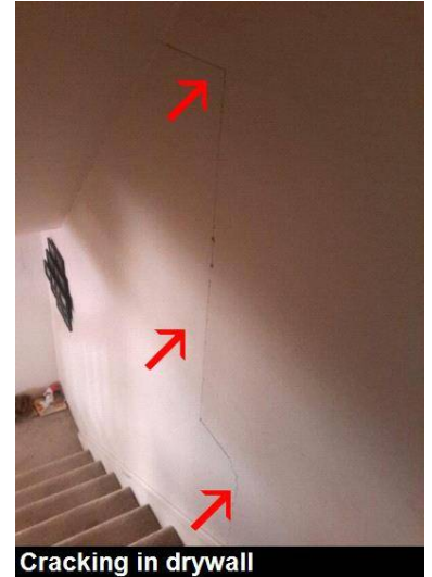
Cracking in drywall
