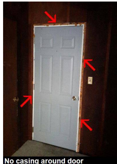
No casing around door
