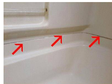
caulk/seal seams in tub areas
