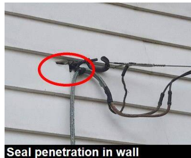
Seal penetration in wall
