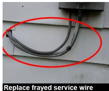
Replace frayed service wire
