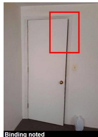
Binding noted at top of the door
