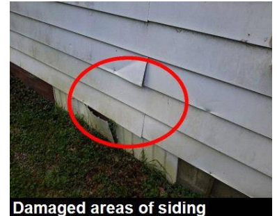
Damaged areas of siding
