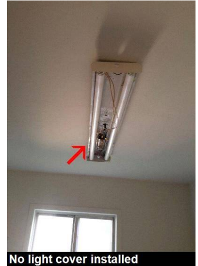
No light cover installed
