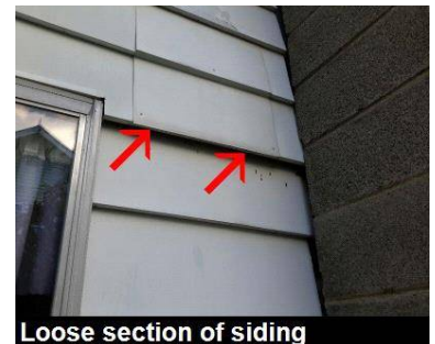
Loose section of siding
