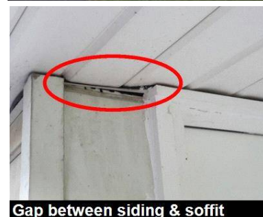
Gap between siding & soffit
