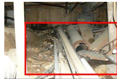
Crawl space is damp without vapor barrier
