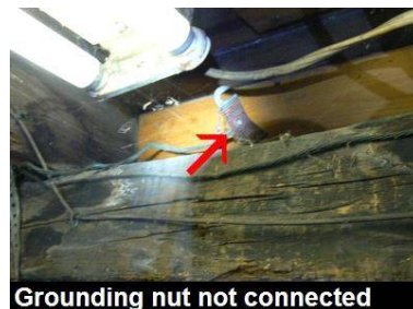
Grounding nut not connected
