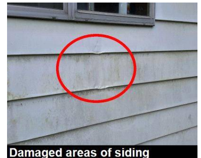
loose/damaged areas of siding
