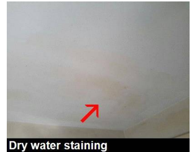
Dry water staining
